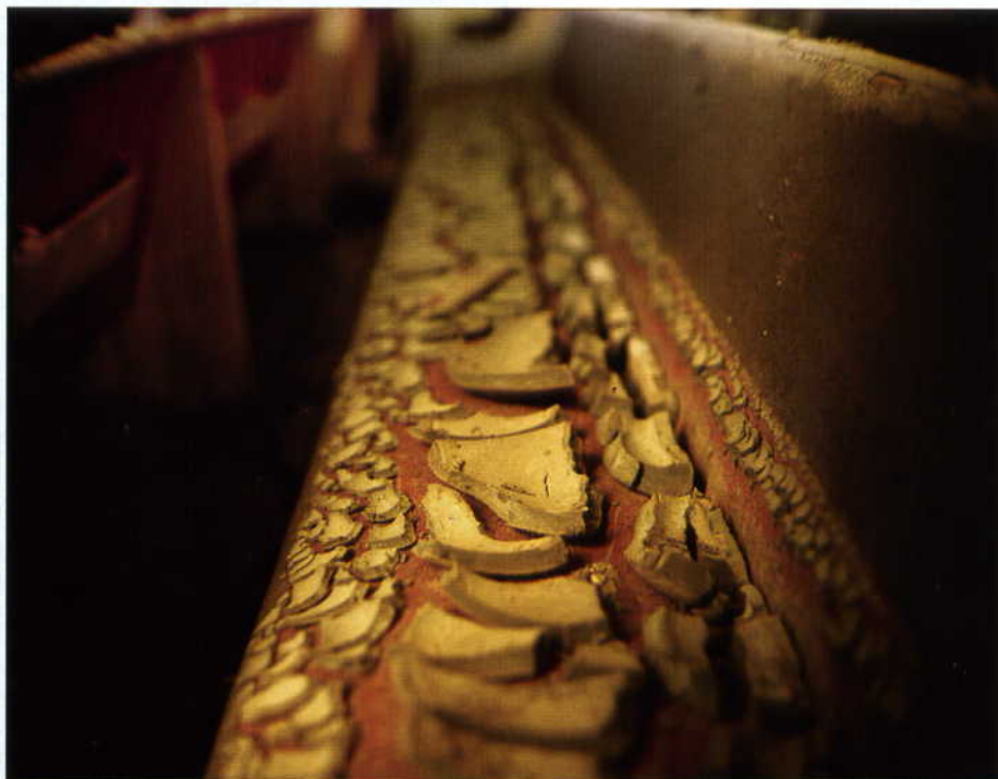
New Orleans Cracked mud upholsters the pews of the Greater St. Rose Baptist Church in the Lower Ninth Ward, where water rose more than 12 feet after the Industrial Canal levee failed.
